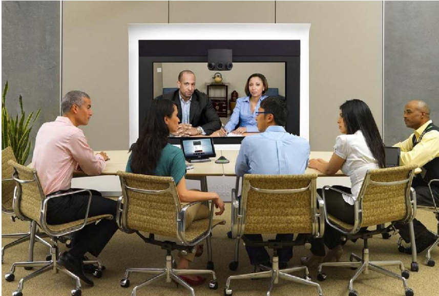
Figure 2. Cisco TelePresence TX1310 65
